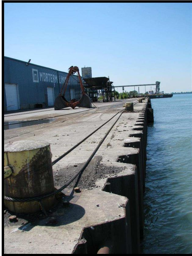
Photo 13: Morterm Limited sheet pile wall facing south towards ADM Windsor Grain
